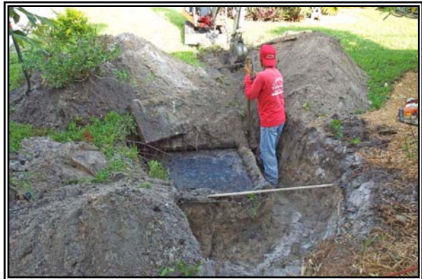
Septic System Repair
