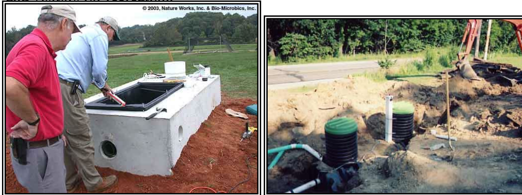
Alternative On-site Sewage Disposal System
