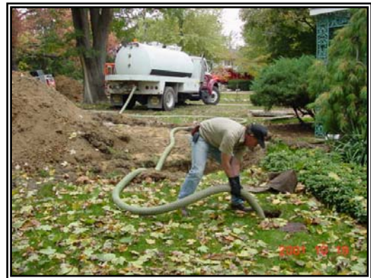
Septic System Pump-out
