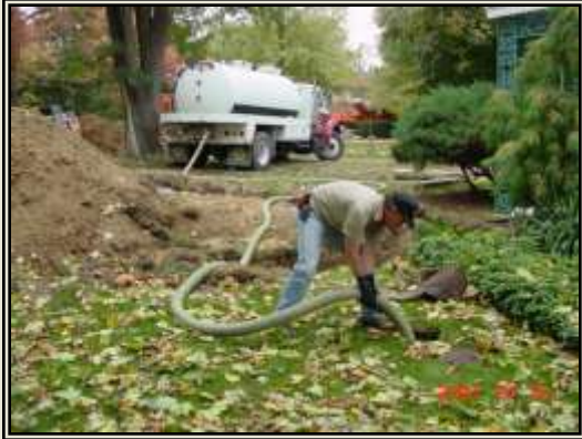
Septic System Pump-out
