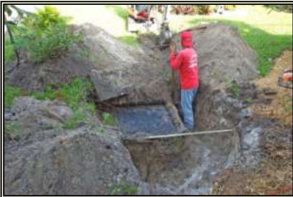
Septic System Repair
