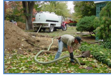
Septic Tank Pump-out
