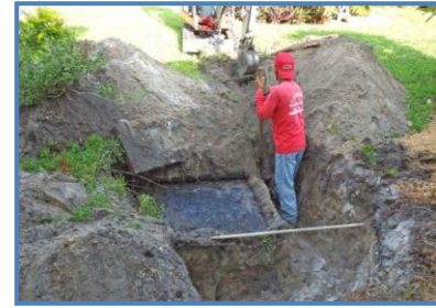
Septic System Repair
