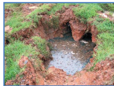
Straight Pipe & Failing Septic System
