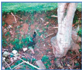
Straight Pipe & Failing Septic System
