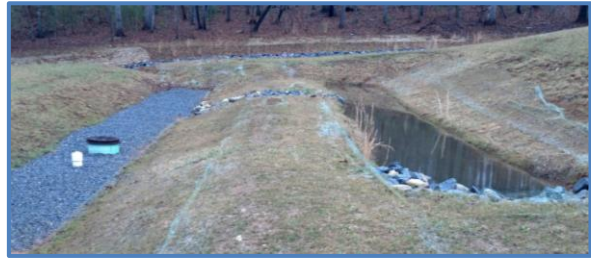
Stormwater Runoff Control Structure
