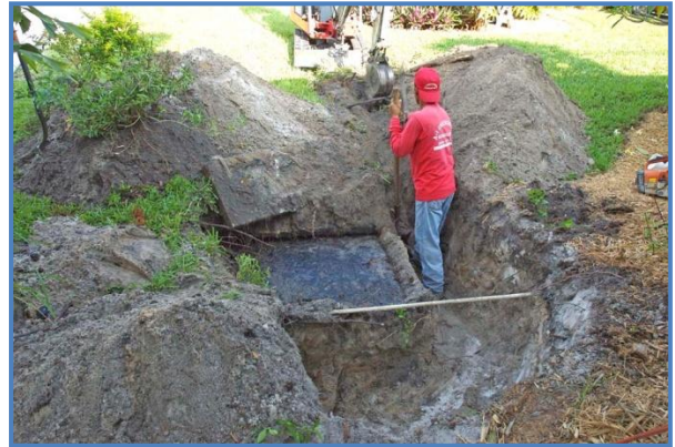
Septic System Repair
