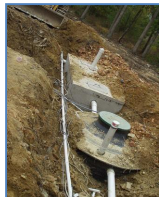
Alternative On-site Sewage Disposal System
